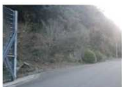
落石防護柵 L = 51.0m
